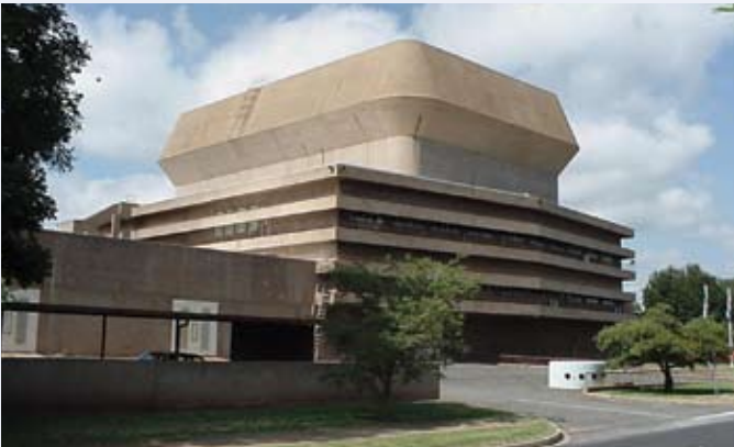
The SAFARI-1 research reactor building
