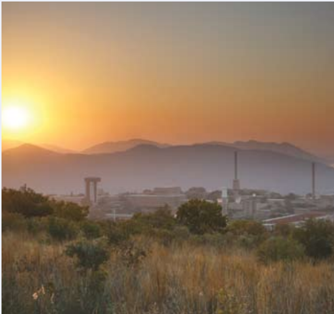
The Necsa site at Pelindaba
